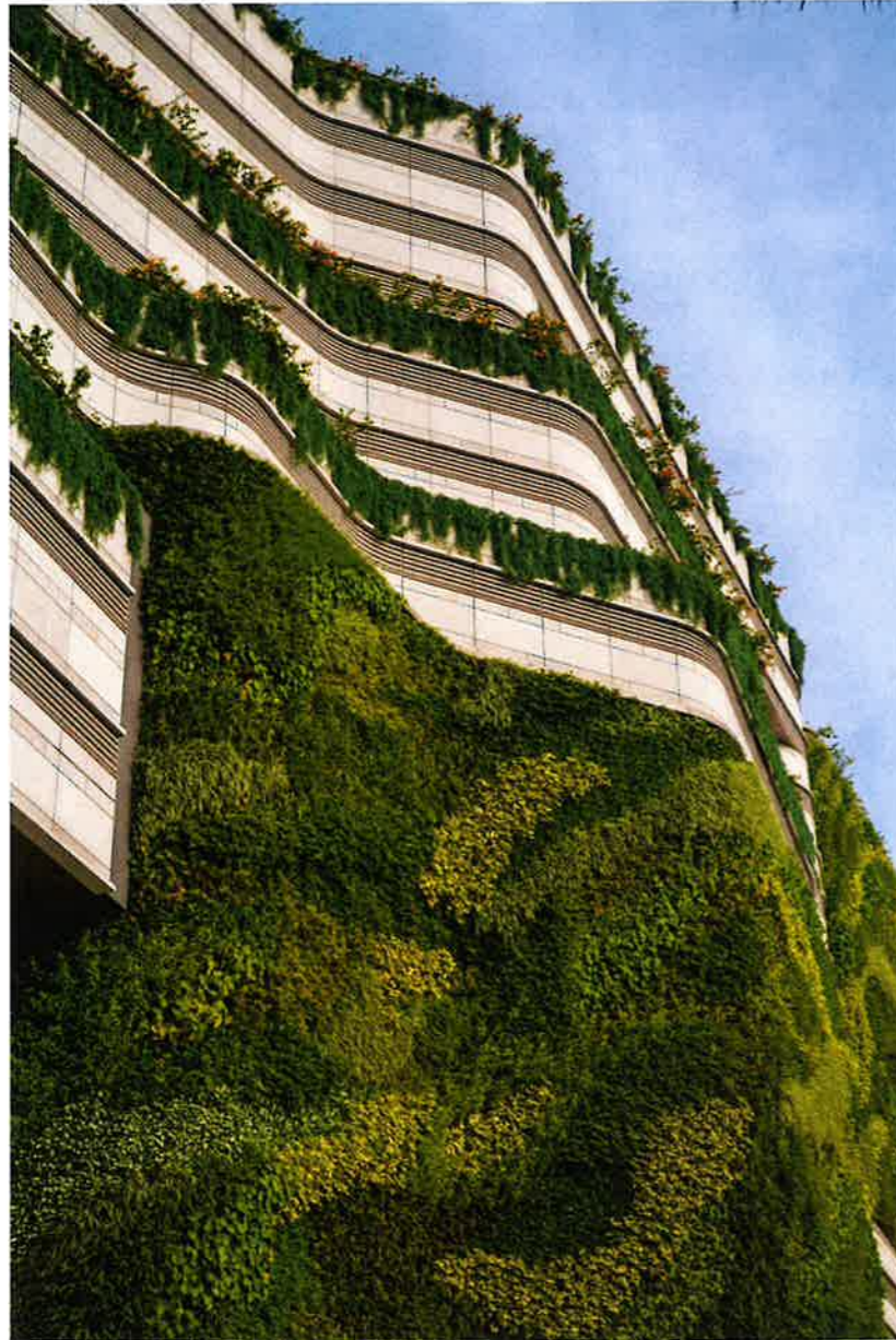
Example of Vertical Greenery
